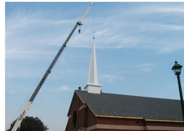
Erecting the 50' foot steeple
